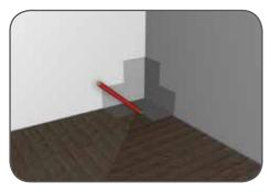
Temporarily place the waterproofing internal corners into position and mark around them with a pencil. Once you have marked they can be removed. This is to show where you need to apply the Pro-SEAL tape sealer.
