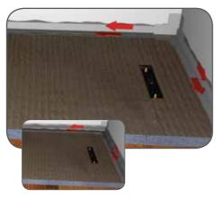
Place the strips of waterproofing tape previously cut in step 8 along the edges of the shower tray, folding half up the wall and half on the shower tray as you go. Press firmly into the Pro-SEAL tape sealer and the tape should also overlap the waterproofing internal corners. When you have finished you can remove the protective gloves and eye and breathing protection.
